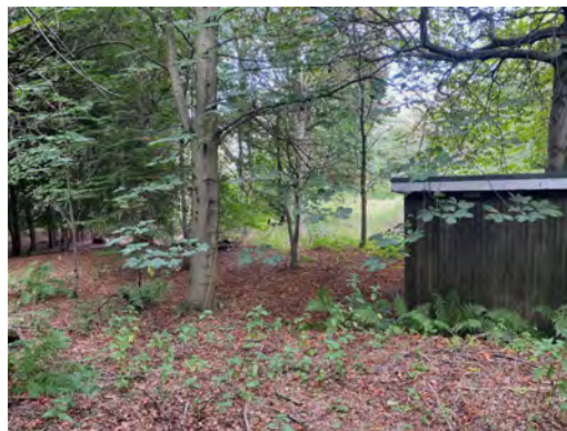
The timber building – south elevation
