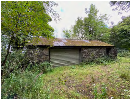
The north building - south elevation
